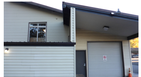
Figure 5 North elevation, west corner
